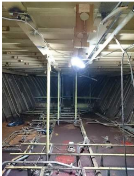
Internal spaces stripped down
