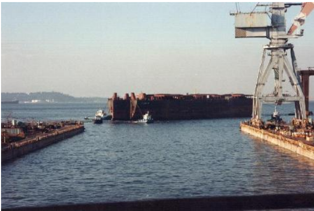
Alianza G1 entering the dry dock
