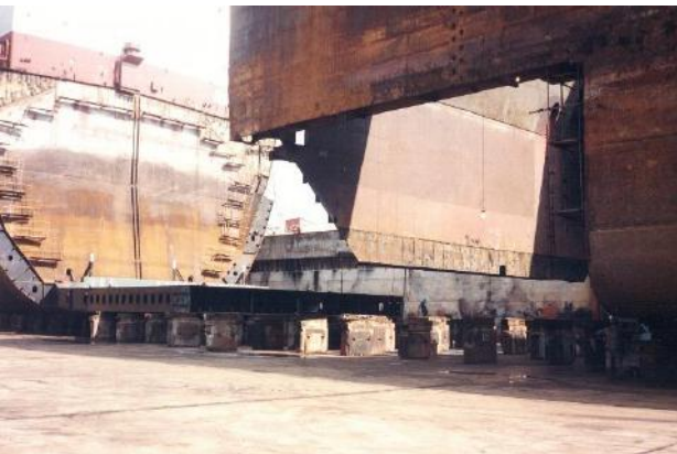
Erecting the transition block
